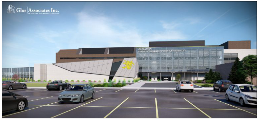
The new Zekelman School of Business and Information Technology occupies the glass section to the right side of the picture. The new modern front of the Student Centre with its geometric design, complete with the St. Clair Griffin, houses the E-Sports arena. The wall of glass windows to the left of the E-Sports arena is 3000 square feet of student space added to the open lab area.
