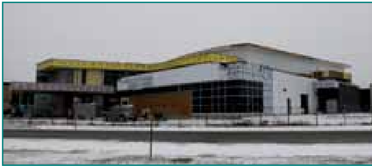
Construction of Thames Healthplex
