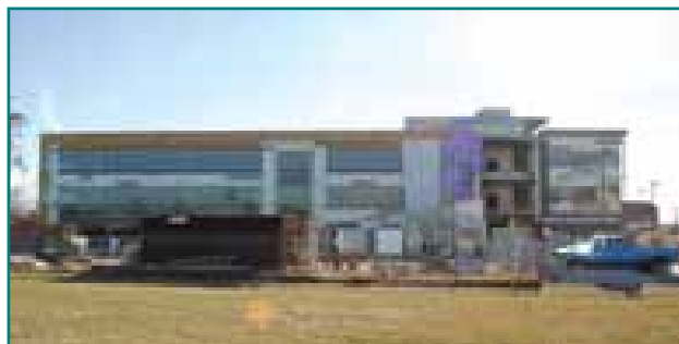
Construction of new Centre for Health Sciences
